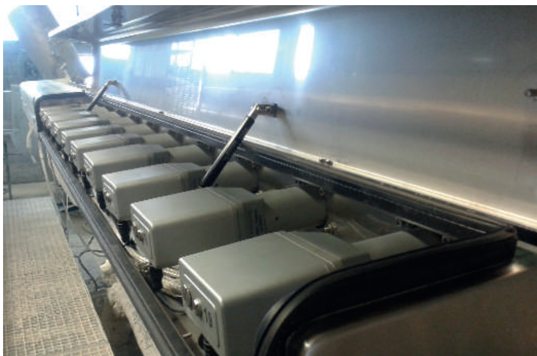
Figure 1. 19 actuators were installed on both the top and bottom sheet sides at Burgo's Sarego mill.
